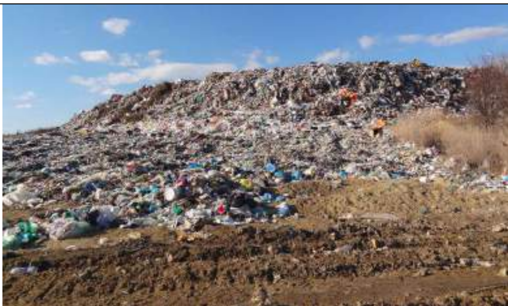
Photo 12: View (from the South border of the site) to North-West direction, the dumpsite area
